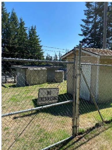
(Above) Pump house and reservoir site
